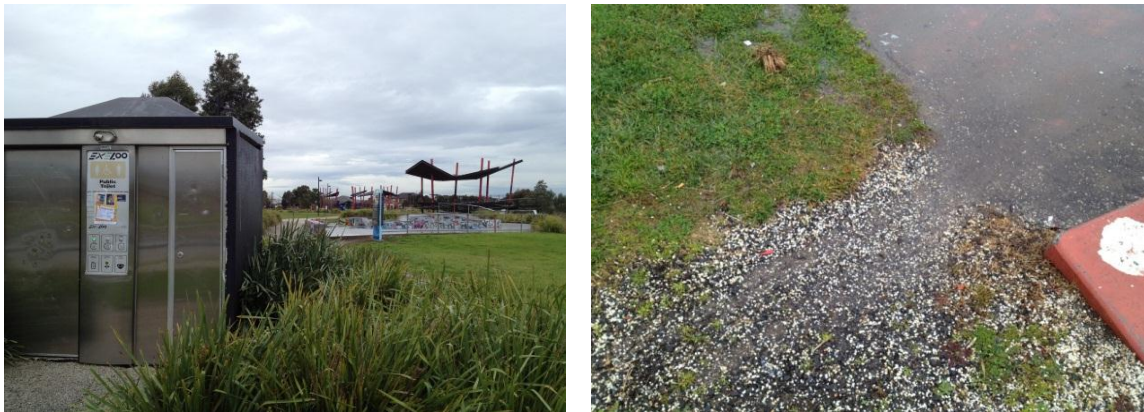
Figure 11: Photos show Exeloo toilet in close proximity to bowl in high profile visual location and Informal path at edge of facility.
