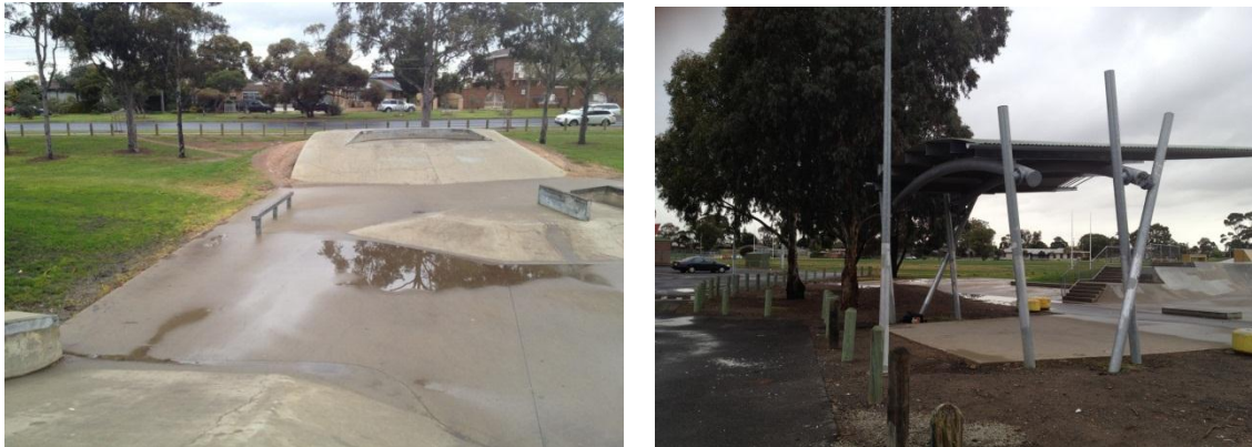
Figure 13: Photos showing significant ponding on the edge of the park and within the riding areas. There are seats and a shelter that provides some amenity for spectators.
