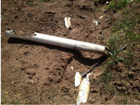
Figure 19: Photo show damaged drainage lines that need repair as part of an ongoing maintenance plan (refer summary below). The other image shows how poor natural surveillance is to this site.
