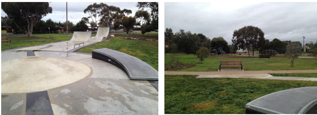
Figure 16: Photos show clean and well maintained facility. The raised end ramps in the background pose a potential hazard. There is also seating and other park infrastructure close to the facility.
