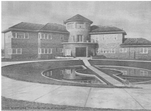
Figure 65 Shirwall Court in Deulgaim Street, Werribee, built for the Carter family in 1937. The house now operates as a nursing home, Mersey Side Health. Source: Lost Werribee Facebook Page
