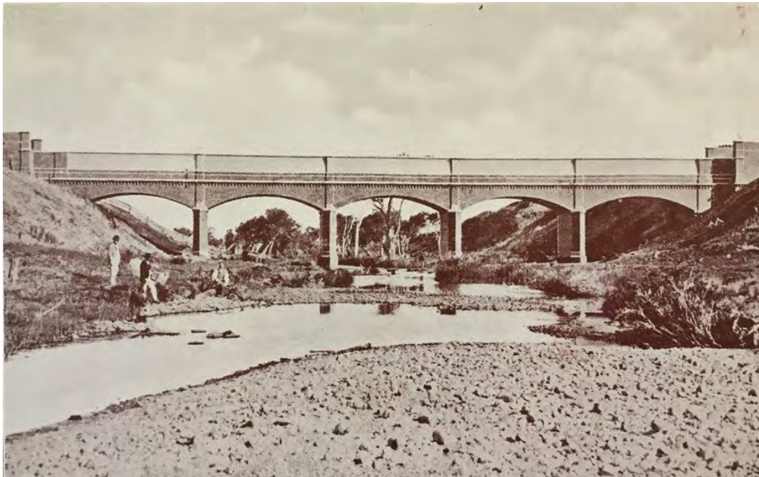
Figure 50 Outfall Sewer, Werribee River Aqueduct, c. 1900s-10s Source: Gibbs 1925
