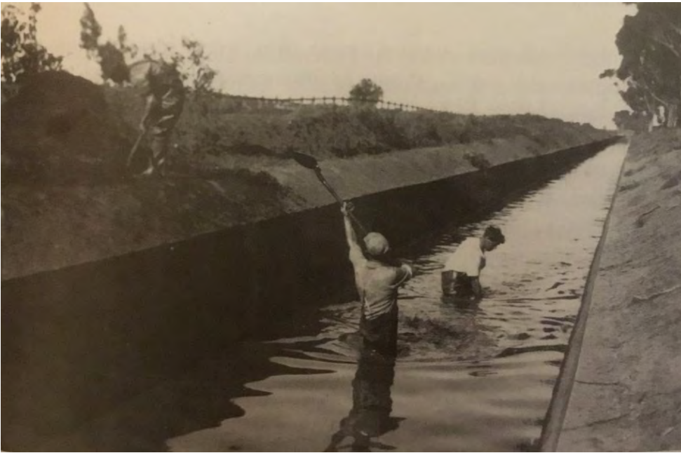
Figure 55 Workers at the Metropolitan Farm, Werribee, cleaning the silt out of the sewerage channels.
