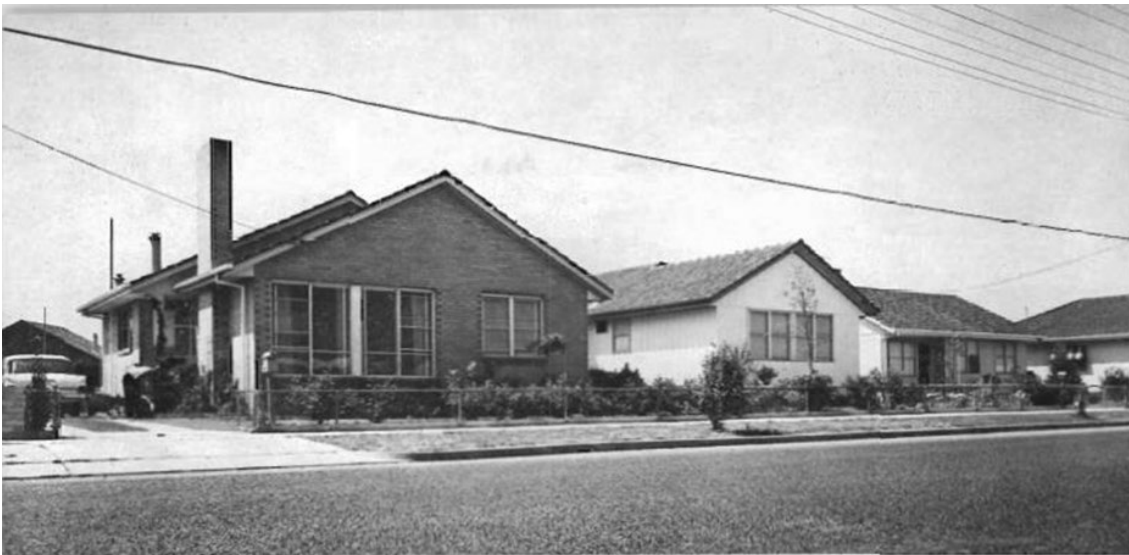
Recently constructed houses at Werribee
