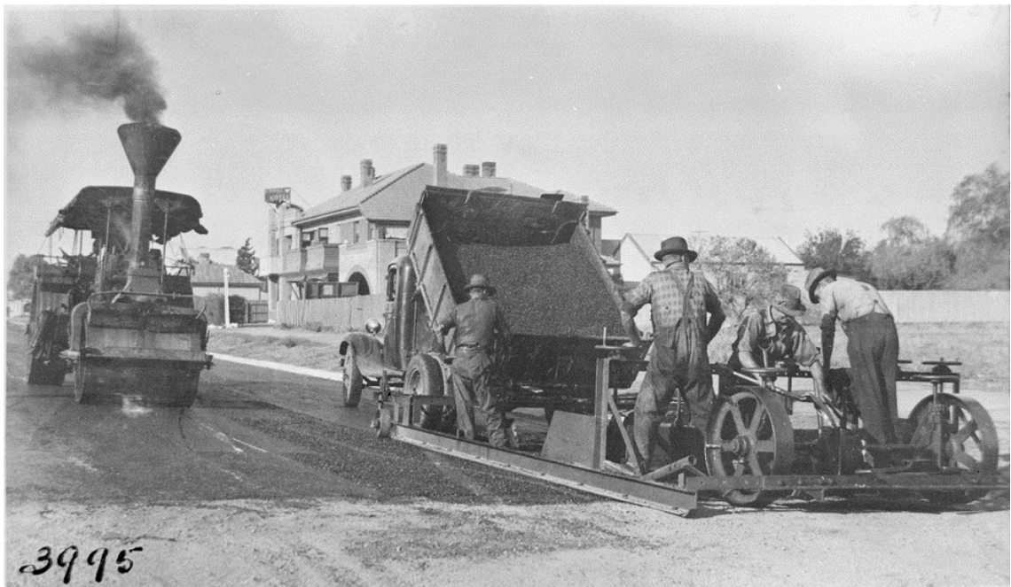
Figure 29 Road workers drag spreading in Werribee township, April 1940, showing the Bridge Hotel in the background.
