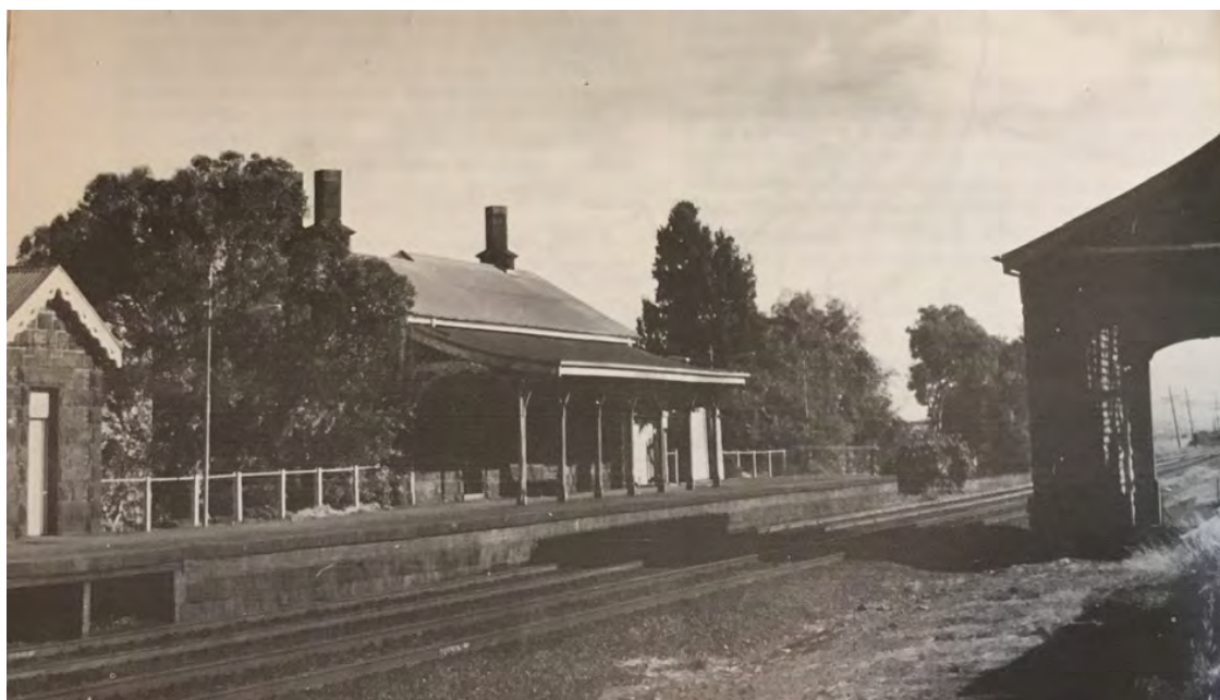
Figure 30 Bluestone railway station and engine shed at Little River, constructed in 1864. Source: Winty Calder, Beyond the View , 1981
