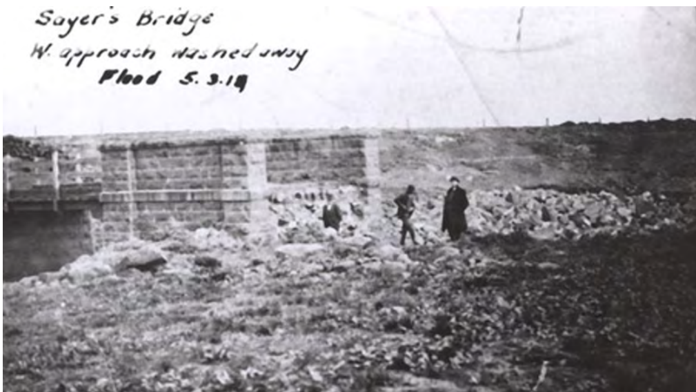
Figure 24 The Sayers Road Bridge following a flood in 1919, where the western approach was washed away. Many of the river crossings and roads in the district were routinely affected by flooding on both the Little River and Werribee River Source: Werribee District Historical Society
