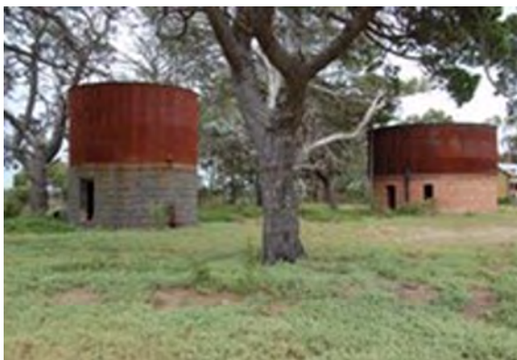
Figure 40 Elevated water tanks on what was formerly Werribee Park, probably c 1870s-80s. Source: private collection
