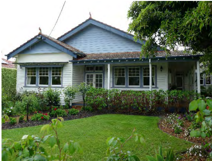
Figure 64 Example of a Californian Bungalow built c. 1920s, Princes Highway, Werribee. Source: Lovell Chen, 2023
