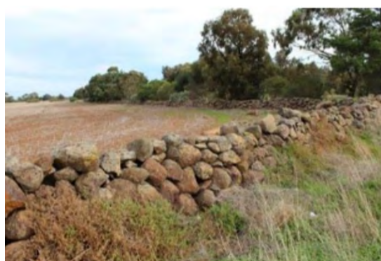
Figure 16 Drystone walls, Old Melbourne Road, Little River Source: Gary Vines, Wyndham Dry Stone Walls , 2015
