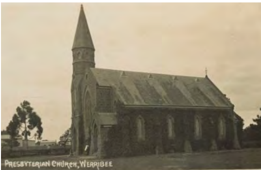
Figure 82 Werribee Presbyterian Church, c. 1911. Source: H96.200/1480, State Library Victoria
