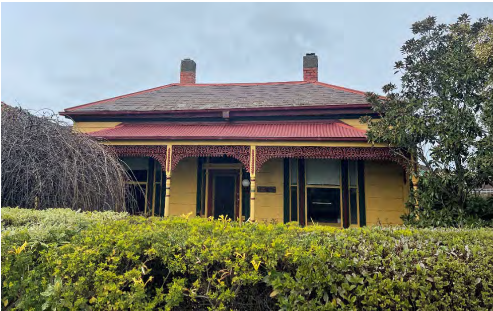
Figure 16 North elevation, fronting Cottrell Street
