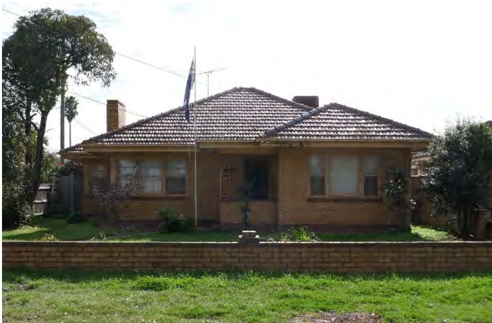
Figure 28 Front (east) elevation
