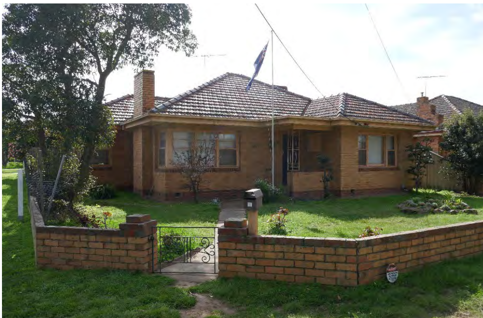
Figure 27 East (right) and south (left) elevations as they present to Geelong Road and Anne Street, respectively
