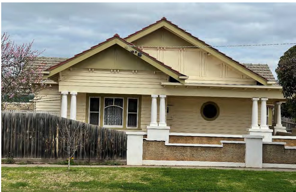
Figure 21 East elevation (Anderson Street)
