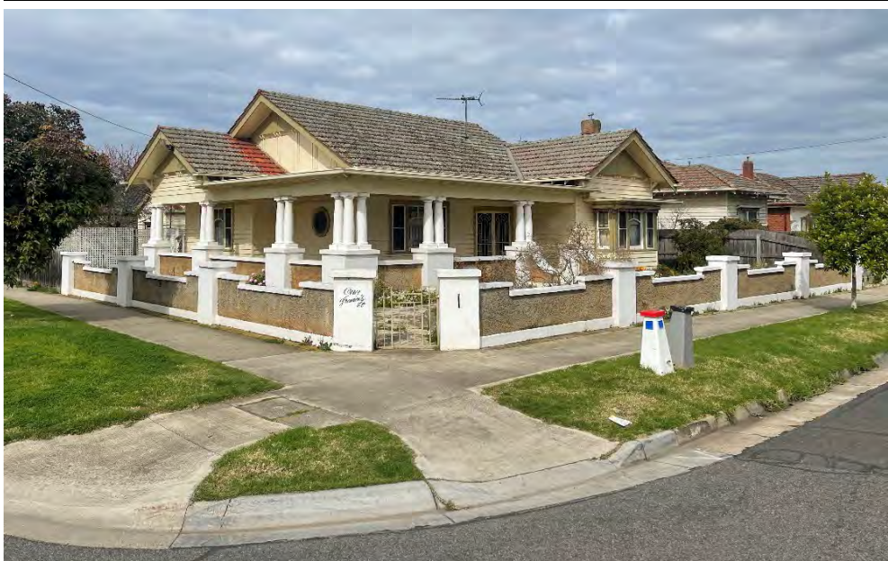
Figure 20 North (right) and east elevations
