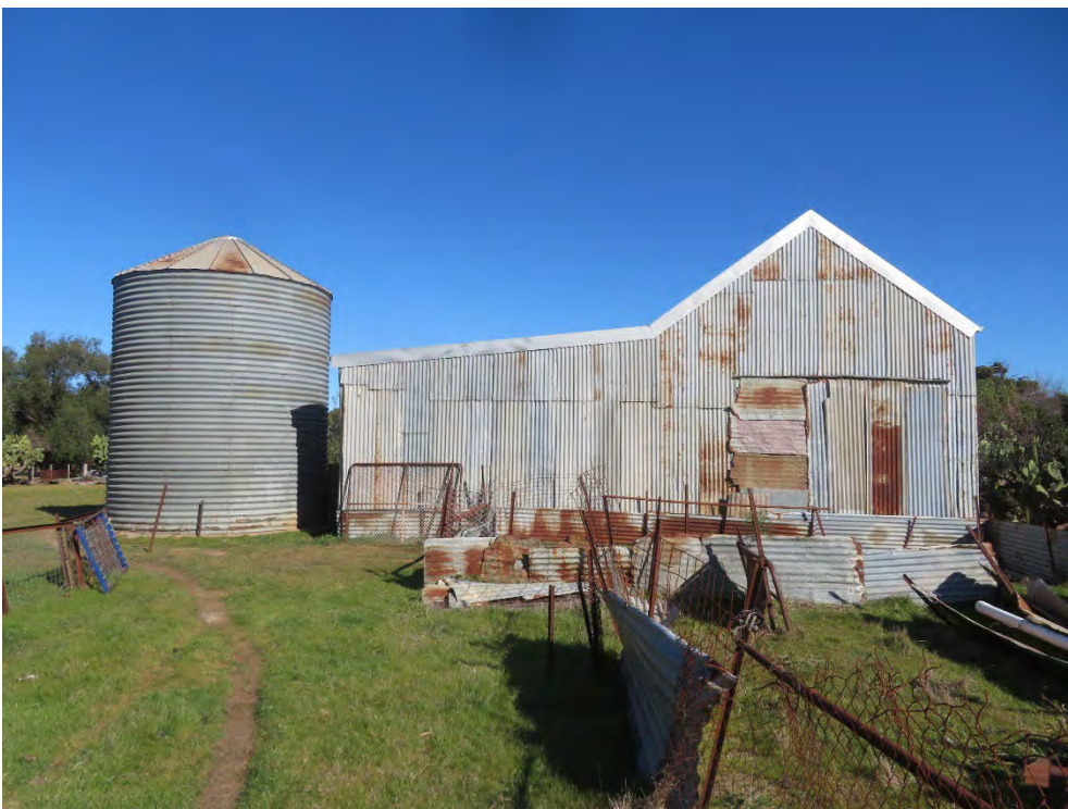
Figure 69 View of farming buildings, including woolshed and grain silo
