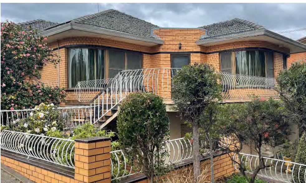
Figure 41 Presentation to the intersection Synnot Street (left) and Purcell Court and
