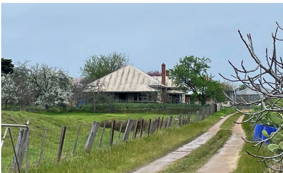
Figure 67 Residence, with steeply pitched roof and chimney visible
