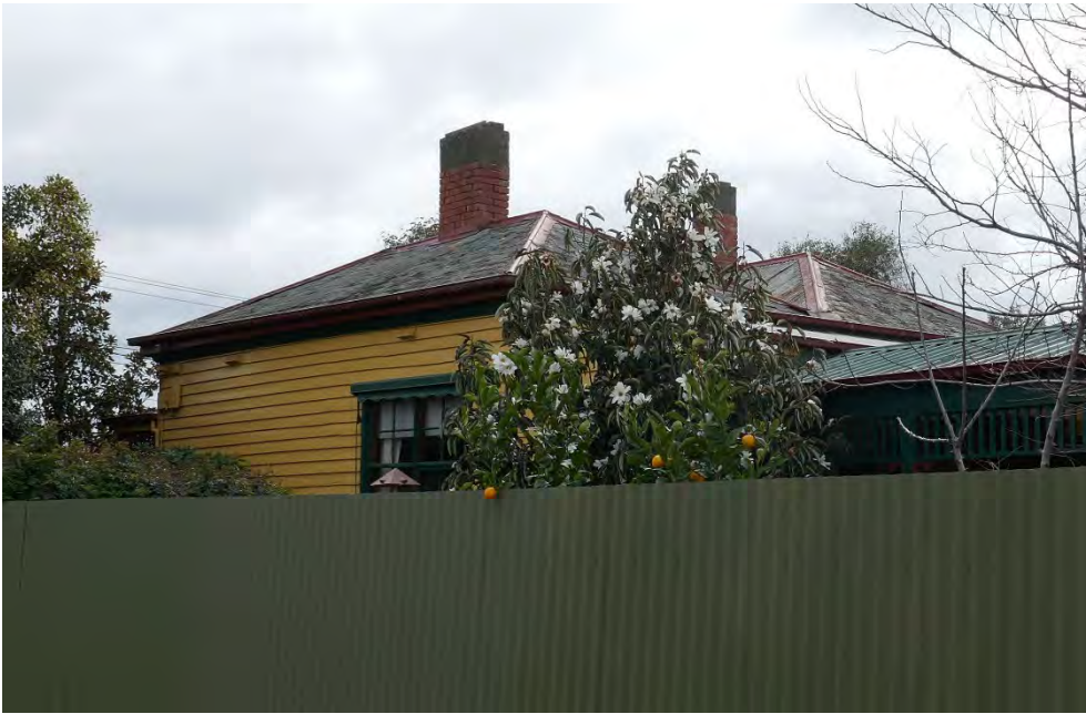
Figure 18 View of the rear of 57 Cottrell Street
