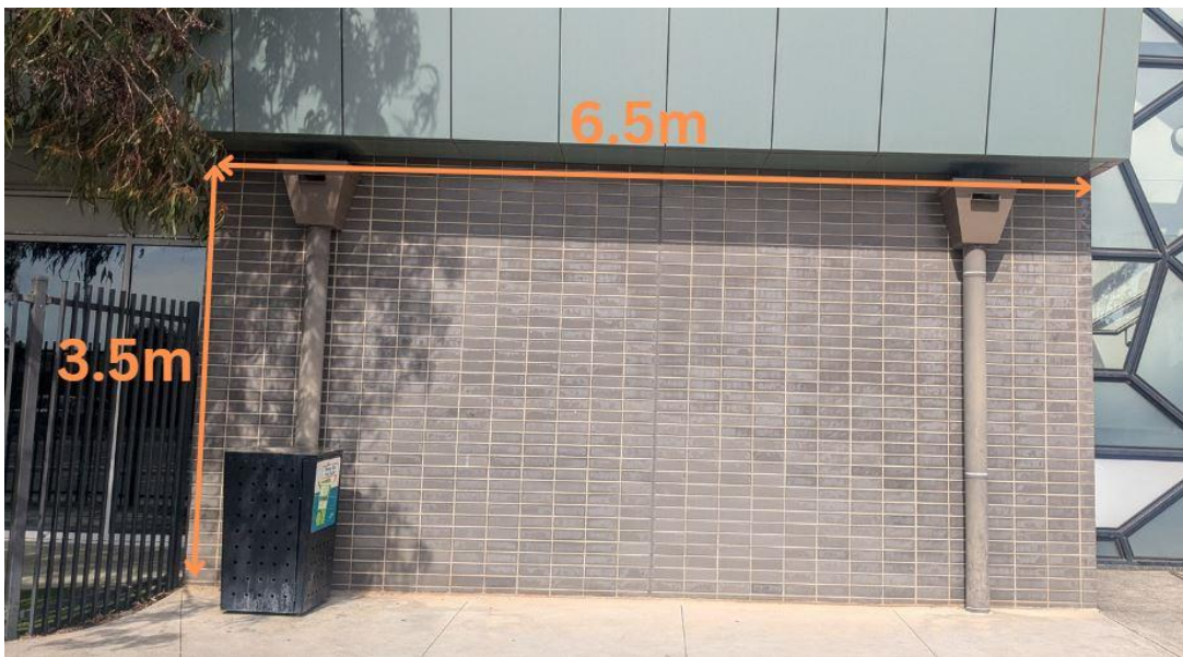
Wall facing Turva Avenue
