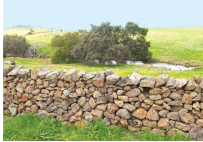
Figure 10 Dry stone wall in natural landscape setting with creek, volcanic cone and red gums, Plumpton.
