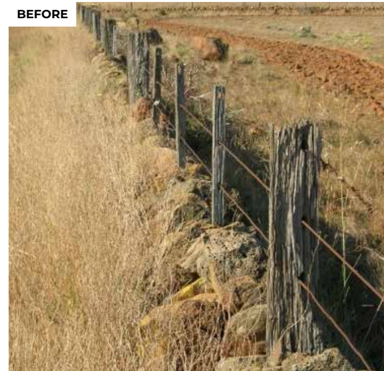
Figure 27 Wall N234 in 2007 before development.
