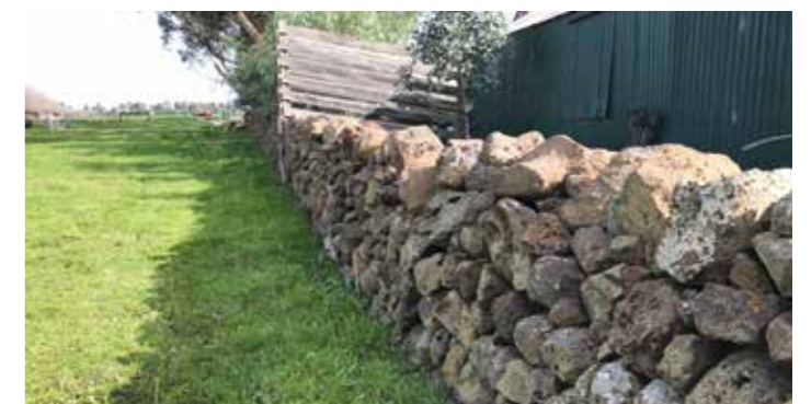
Figure 3 Stone stockyard wall in Toolern Vale. Source: Sera-Jane Peters
