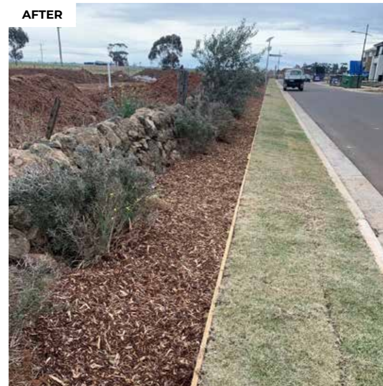
Figure 28 Wall N234 in 2023 after development showing new landscape reserve and retained tree violet.
