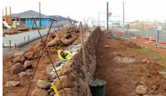
Figure 20 Reconstructed dry stone wall with 2.5m landscape reserve on both sides.
