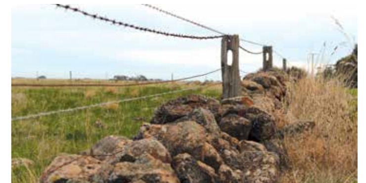
Figure 2 Post and rail composite stone wall in Little River. Source: Wyndham City Council
