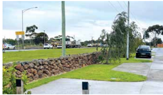
Figure 18 Wider road verge with kerbless parking bays, Wyndham.
