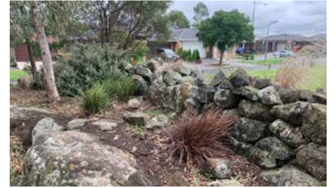
Figure 12 Unrepaired dry stone wall with original vegetation and large trees close to the wall, Epping.
