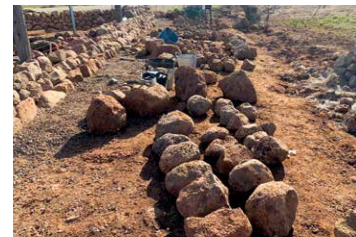
Figure 16 Dry stone wall under reconstruction on Beattys Road, Plumpton.
