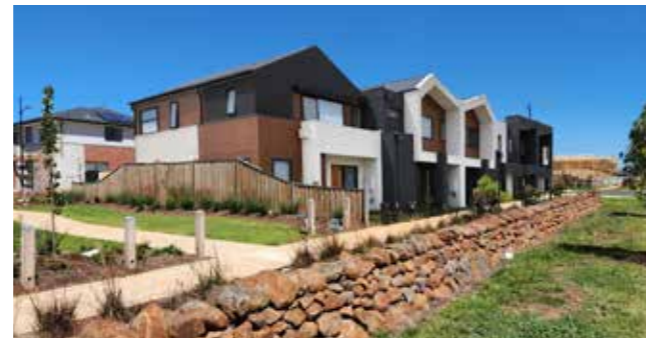
Figure 7 Lots with rear vehicle access on Elliottdale Walk, Rockbank. Source: City of Melton
