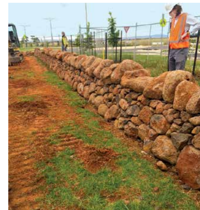
Figure 24 Council officer and developer evaluating dry stone wall reconstruction.
